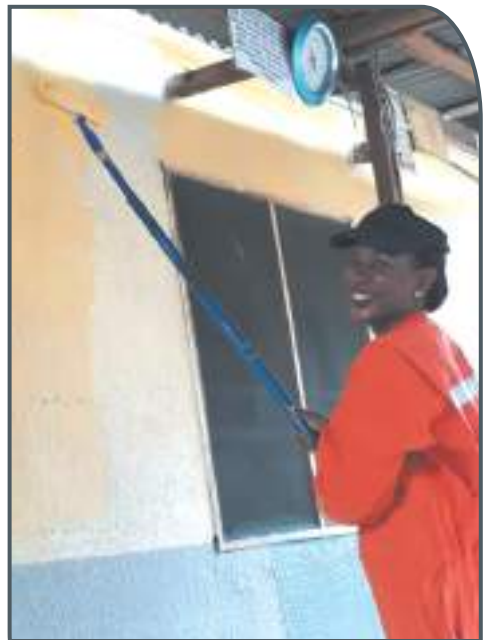
GSK employee happily repainting the GSK House at SOS Village
